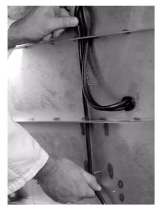
**Step 11:** Install the green ground wire to the back of the switch box using a 5/16" nut driver.
