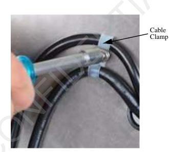
**Step 10:** Install the green ground wire to the panel.
