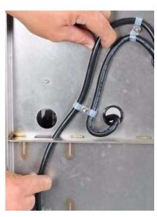
**Step 11:** Install the green ground wire to the back of the switch box using a 5/16" nut driver.
